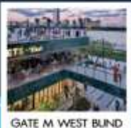
GATE M WEST BUND
